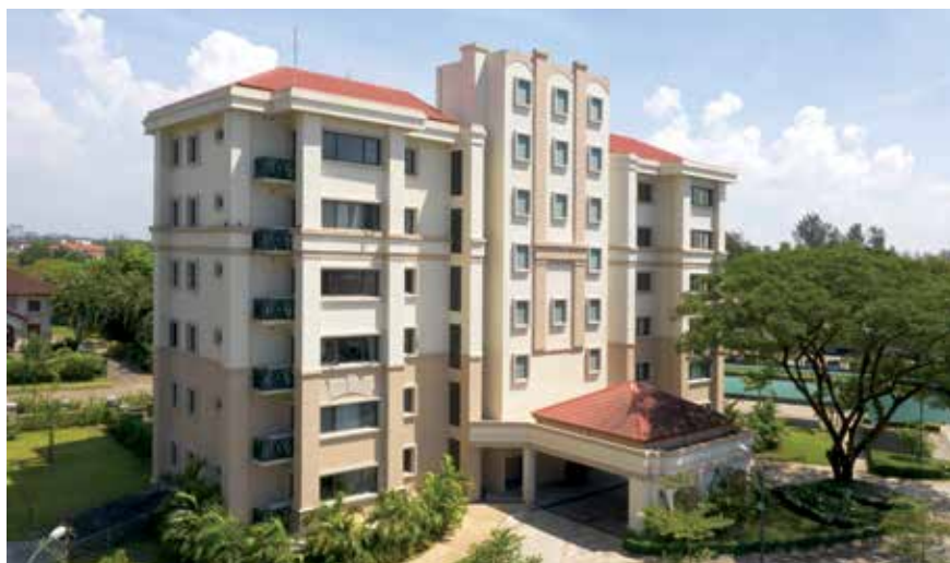
A Golf Apartments, a 24-units residential development for lease at Pun Hlaing Estate.
